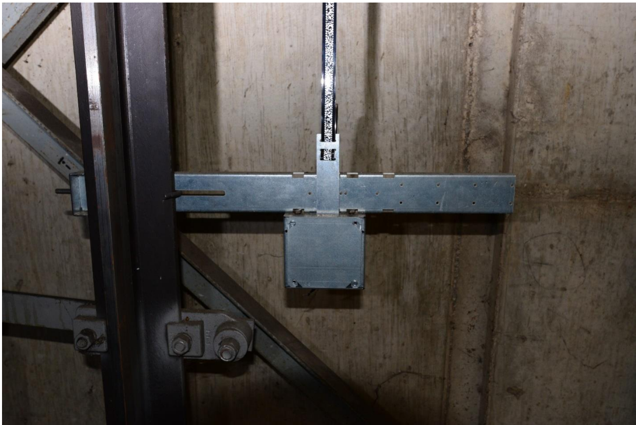
Figure E1.4: Bottom Tape Bracket
