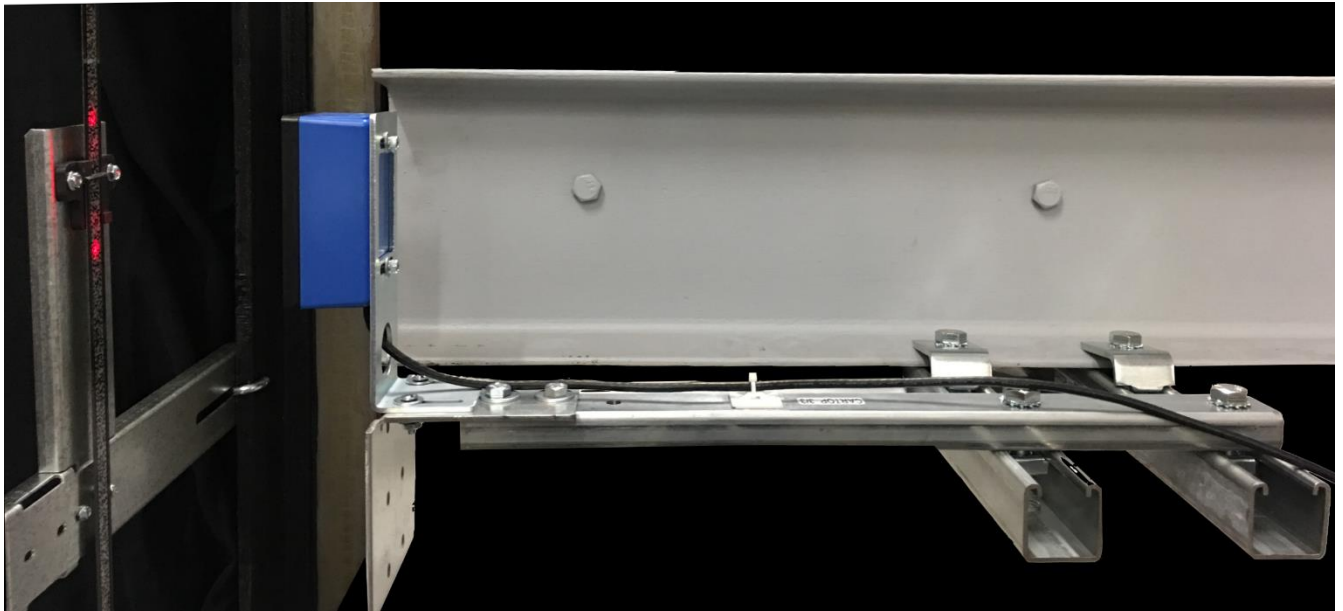
Figure E1.7: CEDES APS Camera Mounting Bracket
