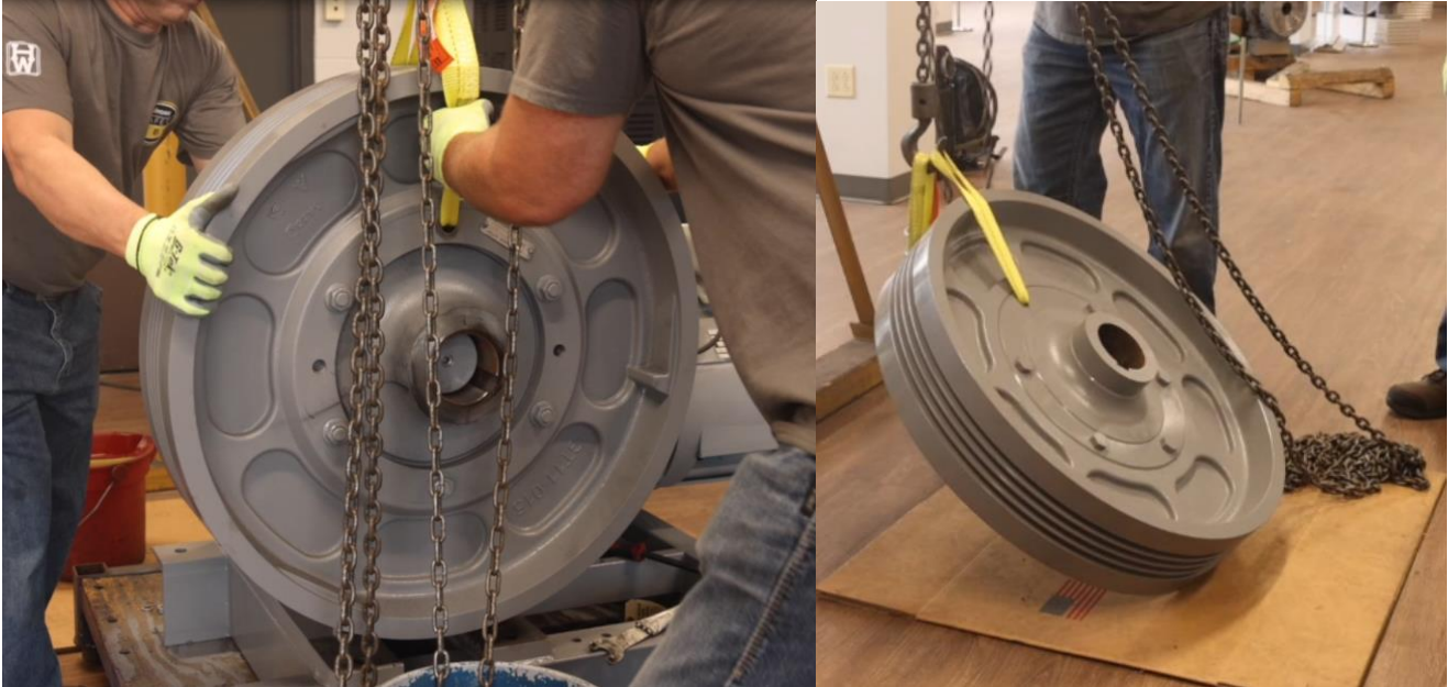
Figure 4-26: Remove Traction Wheel From Shaft and Lay On Floor In Orientation Shown
