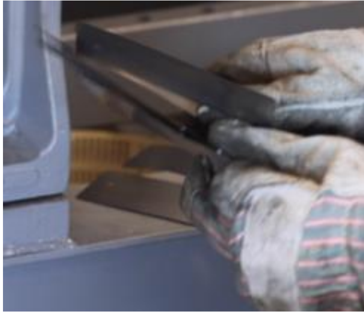
Figure 4-157: Add More Shims to Shim Pack To Achieve Required Indicator Reading
