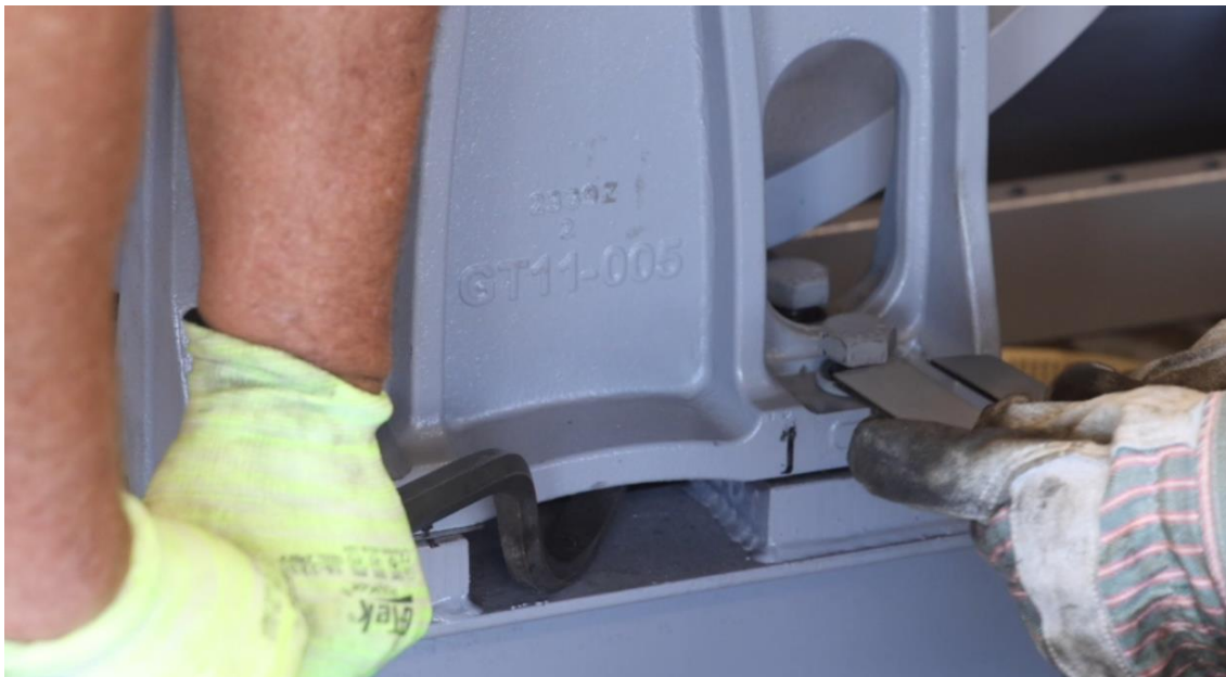
Figure 4-108: Pry Outboard Stand Up to Insert Thicker Shim Pack
