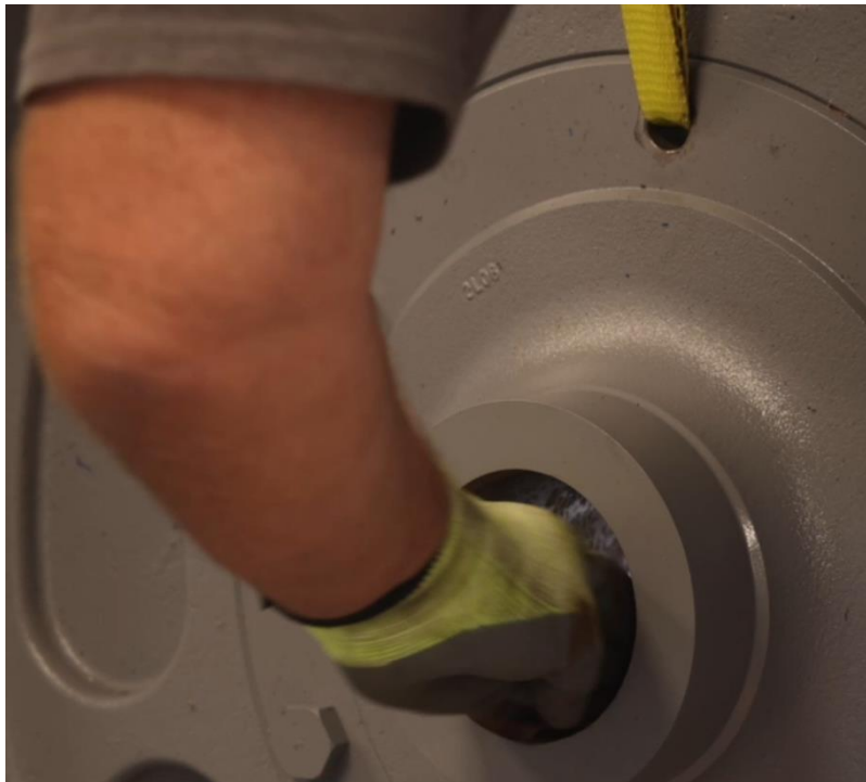
Figure 4-137: Thoroughly Clean Bore of Traction Wheel Hub
