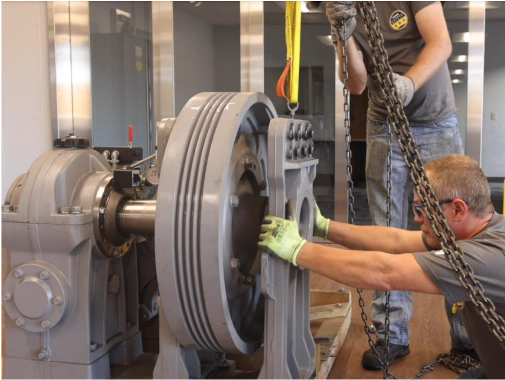
Figure 4-145: Install Outer Outboard Stand Over Bearing
