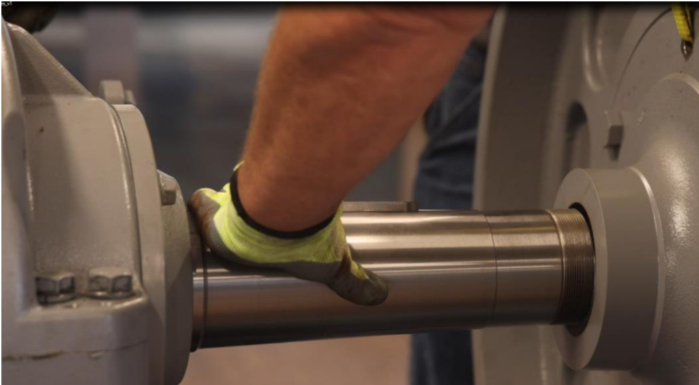
Figure 4-90: Hoist the Traction Wheel to the Shaft
