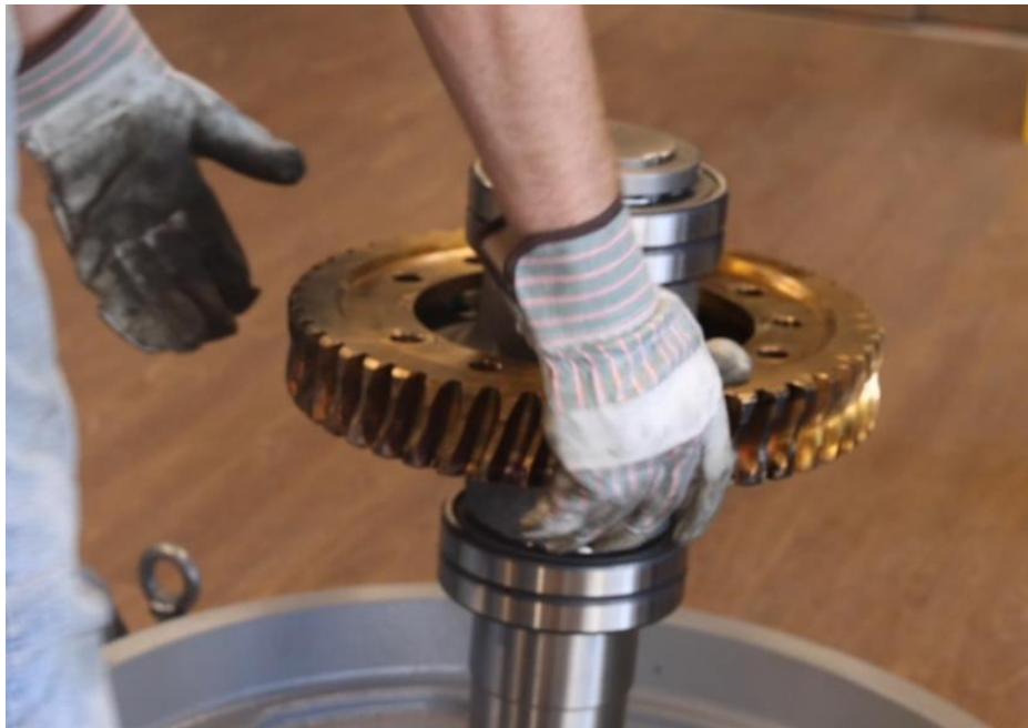
Figure 4-53: Place Bronze Gear on Gear Hub
