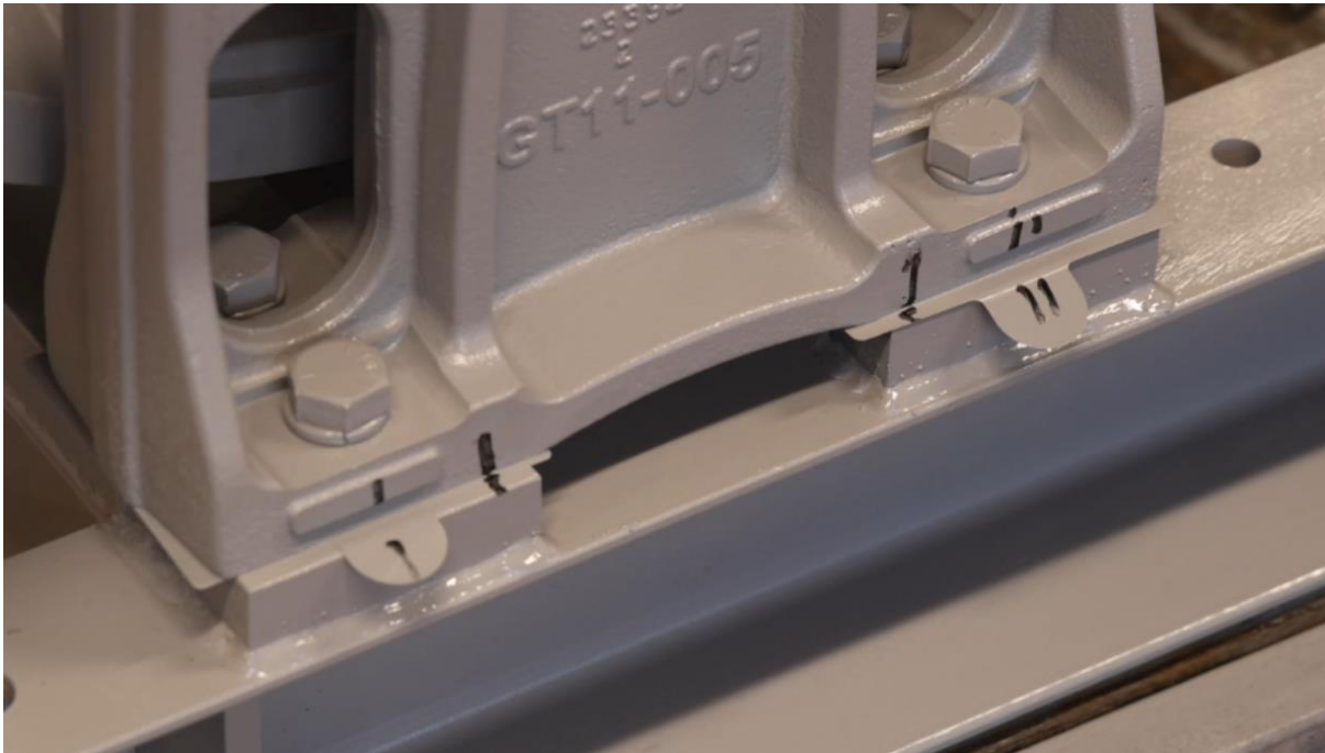
Figure 4-5: Marked Positions of Shim Packs After Marking
