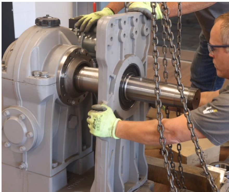
Figure 4-120: Hoist the Outboard Stand to the Inner Bearing
