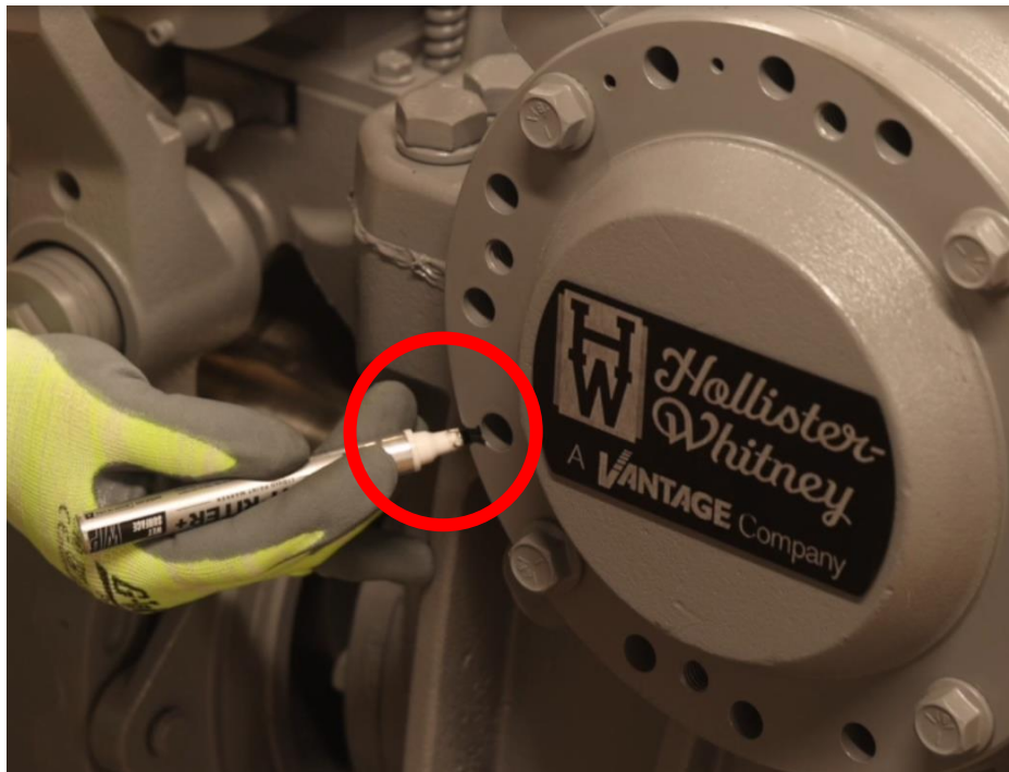
Figure 4-3: Mark Position of Notch In Eccentric onto Lower Housing
