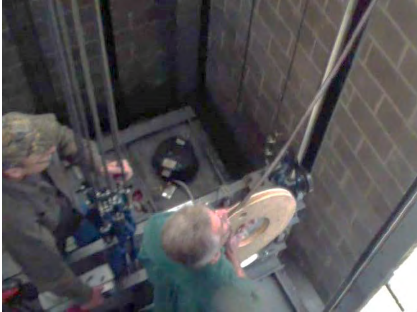
Figure 2-5: Unroll the Encoded Tape
