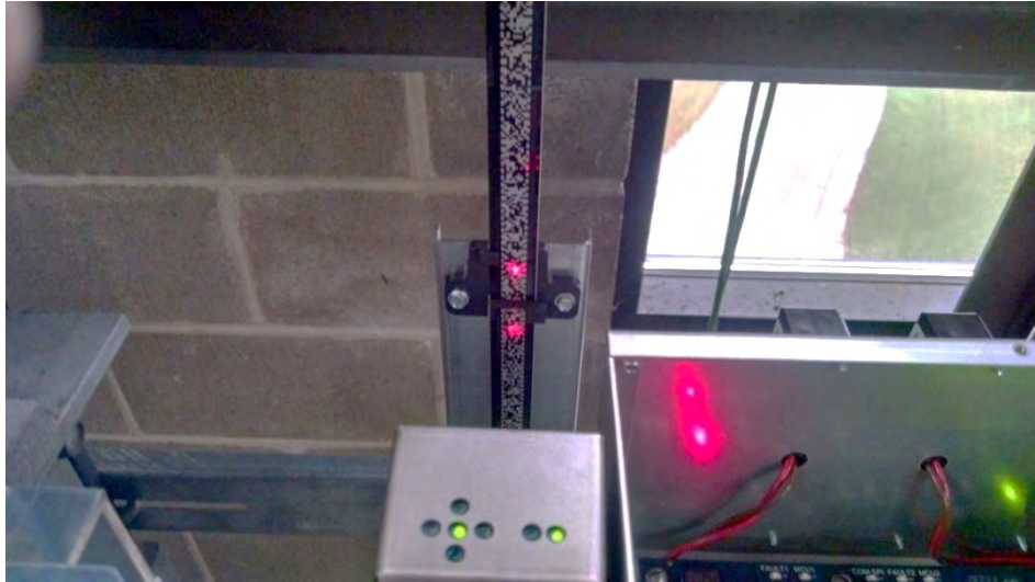
Figure 2-21: APS Selector Alignment Spotlights
