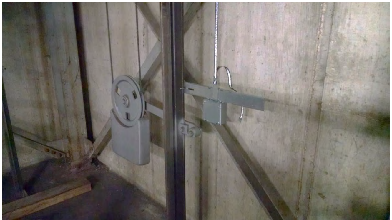
Figure 2-8: Encoded Tape Mounting – Bottom Bracket
