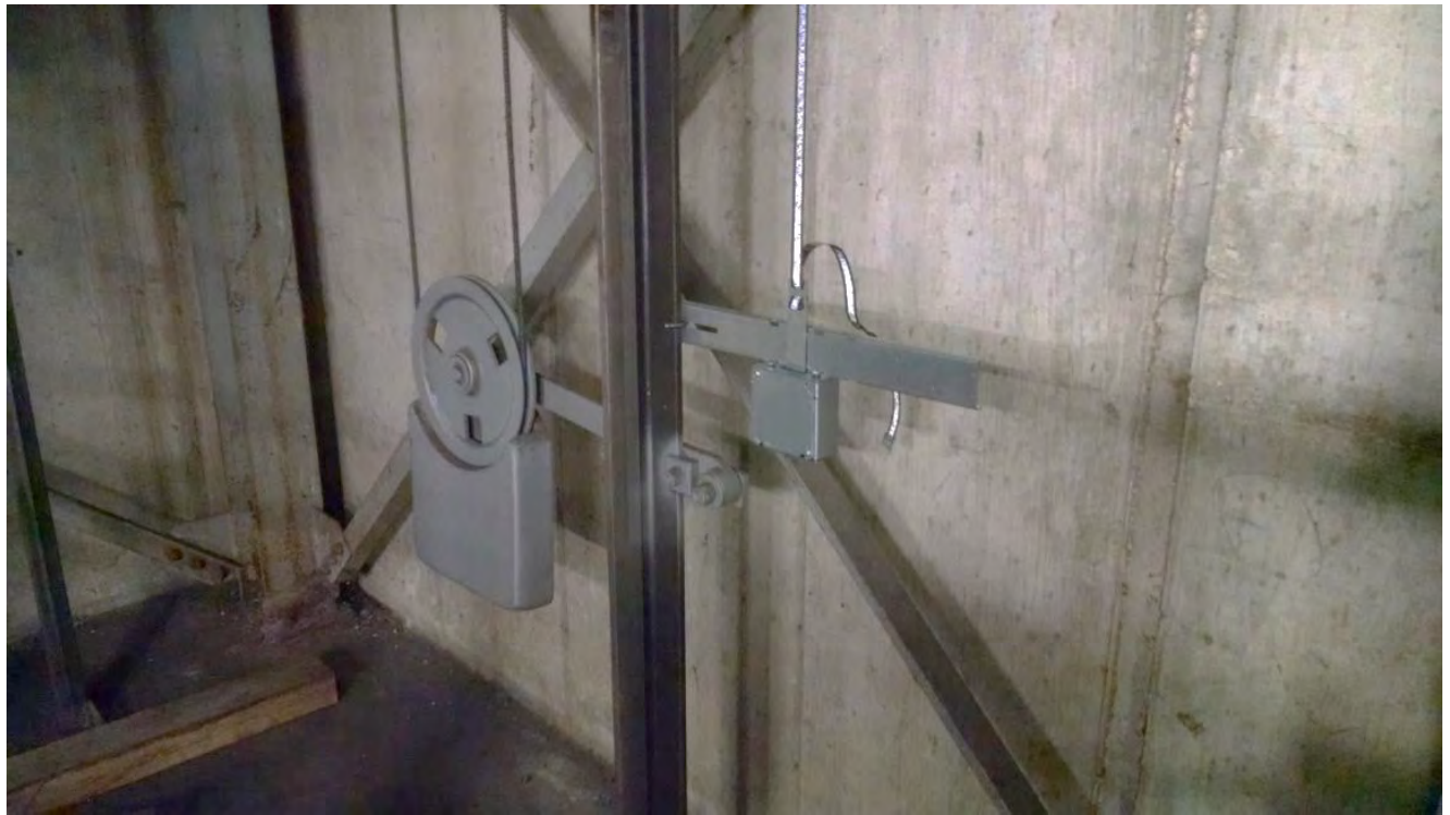
Figure 2-8: Encoded Tape Mounting – Bottom Bracket
