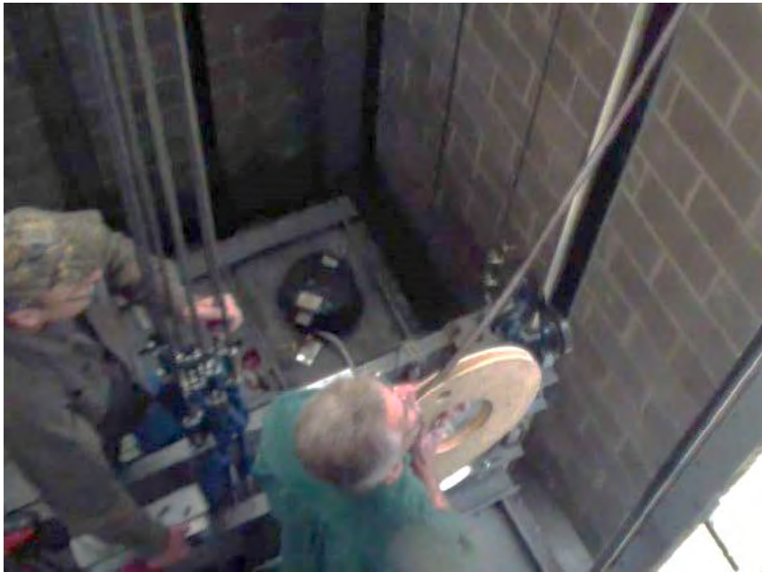
Figure 2-5: Unroll the Encoded Tape
