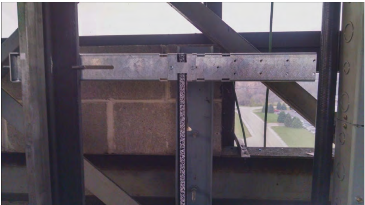
Figure 2-1: Encoded Tape Mounting – Top Bracket
